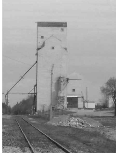
Figure 5- A typical wooden crib elevator at Hudson Bay, SK
