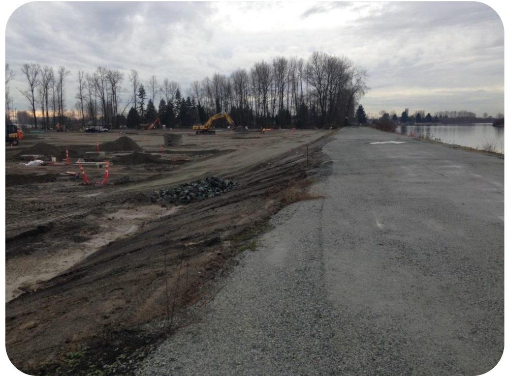
Hamilton Transit Centre Dike Construction
