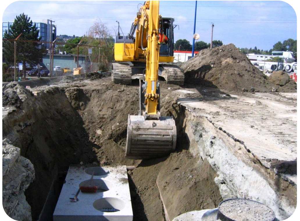
Storm Drainage upgrades with high-flow bypass
