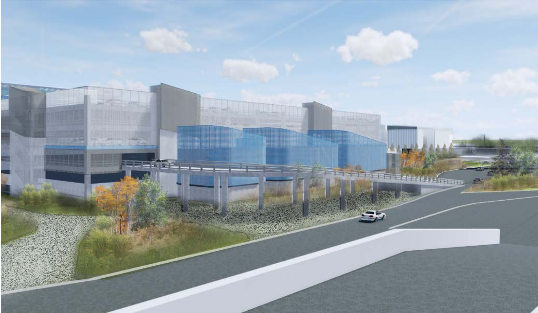
Rainwater Collection System
